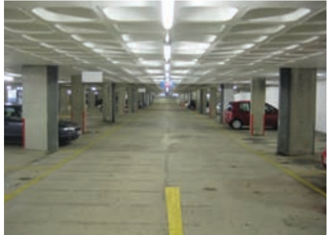
After: Improved lighting levels, lower energy fittings, surfaces blast washed
