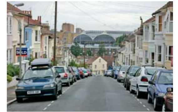
Brighton Station roof from Prestonville
