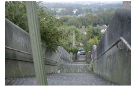
Difficult but distinctive pedestrian link, Tivoli
