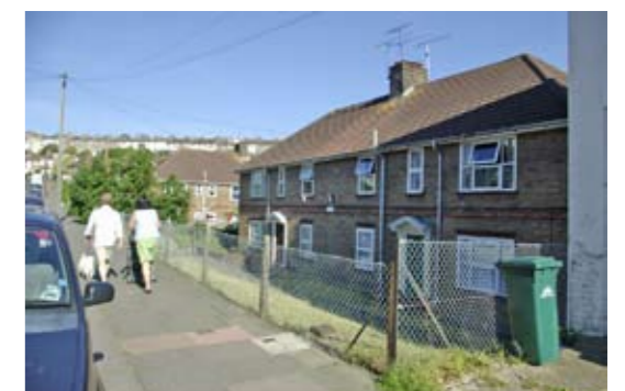
1920s terraced flats, some side-on to street
