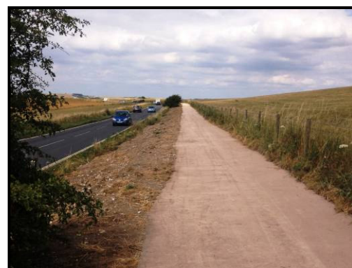
New Woodingdean to Falmer path – under construction
