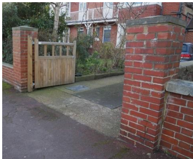
Figure 40 – An existing opening with its widened access. A new pier with a modern wooden gate is evident.
