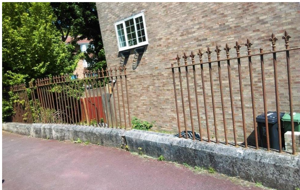
Figure 16 – The railings to the grounds associated with The Attree Villa.
