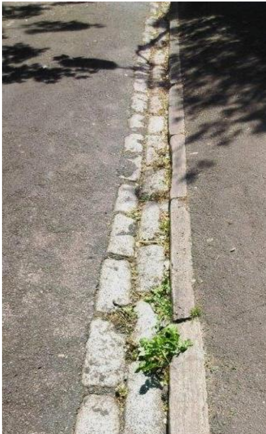
Figure 41 – Purbeck Marble kerbs and limestone setts
