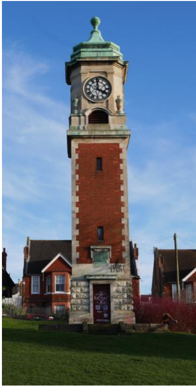
Figure 32 - West elevation, Clock Tower
