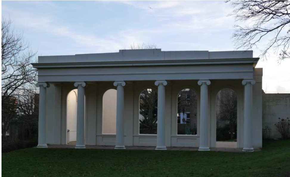
Figure 13 – the surviving North Wall and Ionic Portico of the former Spa.
