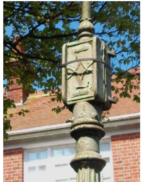
Figure 45 - 1930s BLEECO timer box fitted to a Palmer Green GLS.
