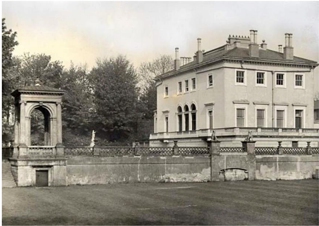
Figure 7 – The Attree Villa, designed by the architect Charles Barry for Thomas Attree.
