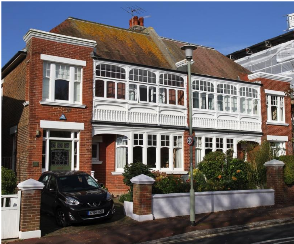
Figure 54 – Nos 12 and 13 West Drive with decorative enclosed balconies.
