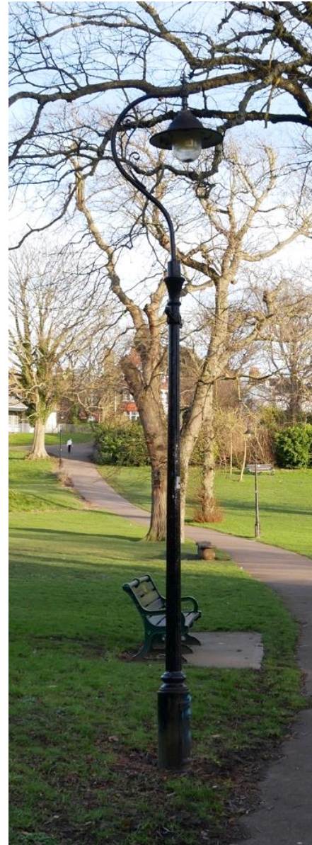
Figure 46 – 47 – Left is an early J. Every, Lewes, electric LS, 1920s, with BLEECO swan neck and ornate 'plinth' base. To the right is a modern cast reproduction column and bracket found in the park.
