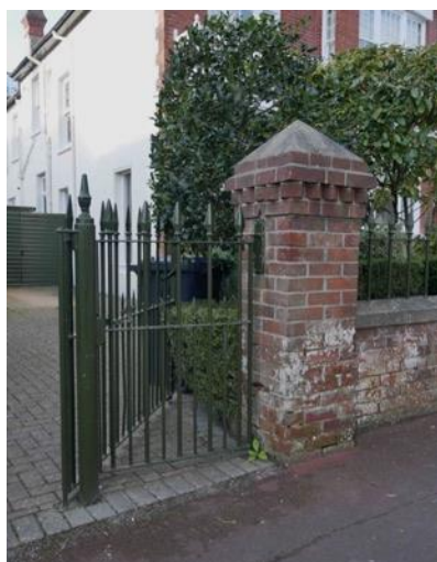
Figure 39– Original walling and pier, gate and vehicular access.
