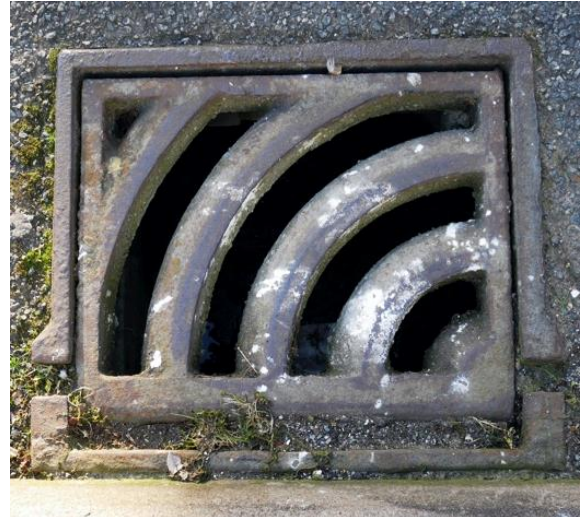
Figure 44 – Modern cast iron grate, Queen's Park Villa
