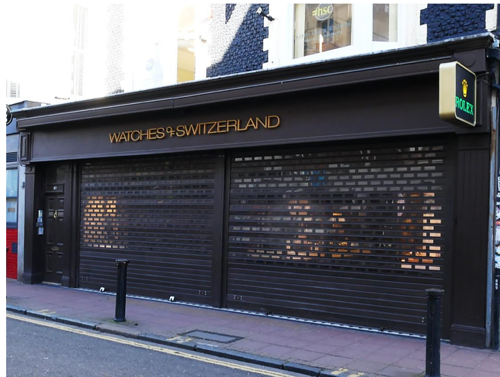
Figure 21 – A partially perforated grille appears largely solid
