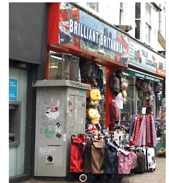
Figure 31 – An ugly equipment cabinet in North Street.
