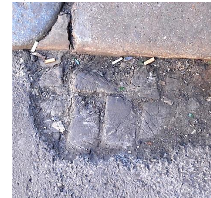
b) Wooden Block to an entrance.
