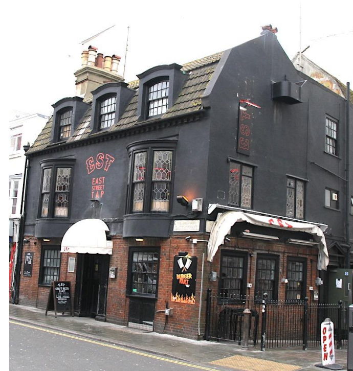
Figure 26 a, b, c – Painted cobbles, dark painted renders to buildings.
