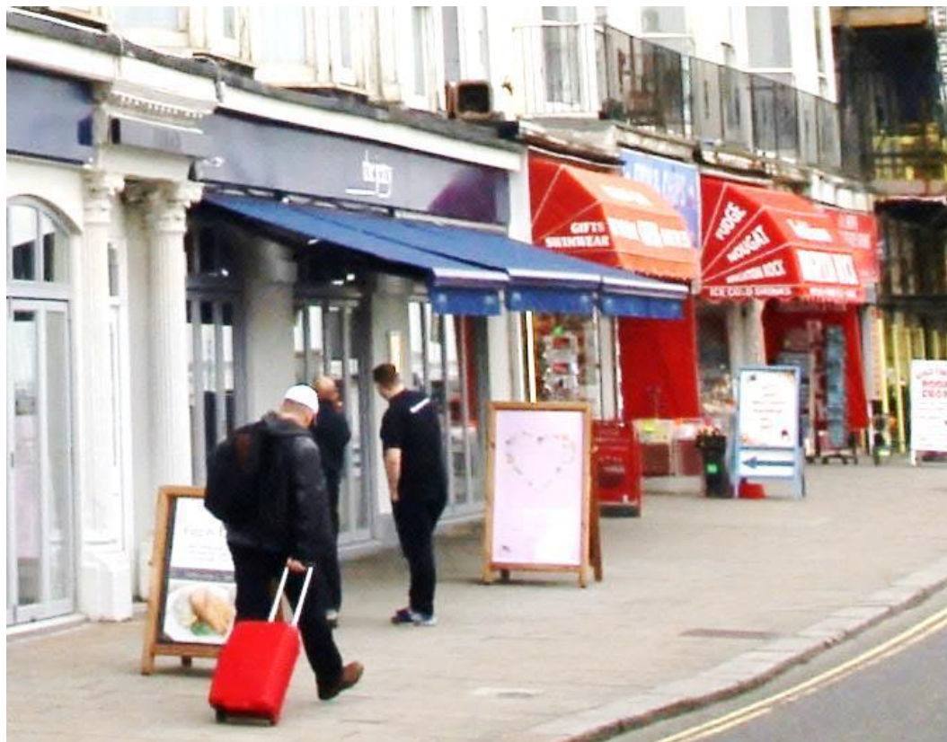
Figure 15 – A traditional roller blind respecting the historic environment alongside inappropriate Dutch blinds emblazoned with text.
