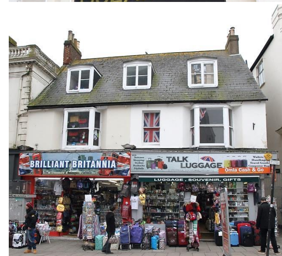
Figure 8 – Shopfronts in North Street failing to respect architectural details.
