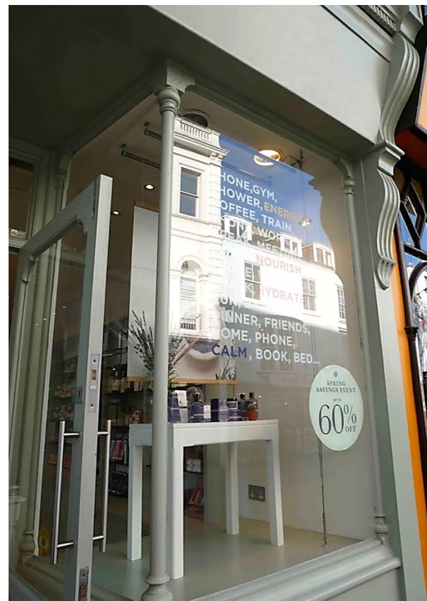
Figure 10 – late 19 th century shopfront.
