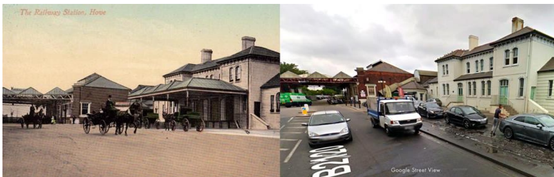
Figure 11 - Hove Station listed Grade II; this includes two station buildings and the footbridge across the railway: The original building facing Goldstone Villas in white render was constructed in 1865-6 in the Tuscan villa style.
