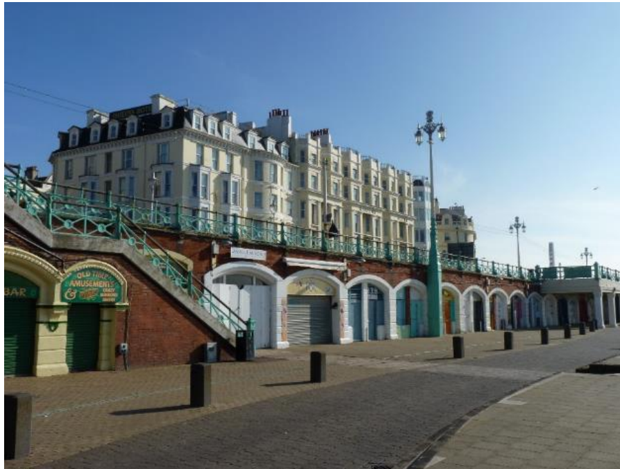
Brick arches supporting King's Road
