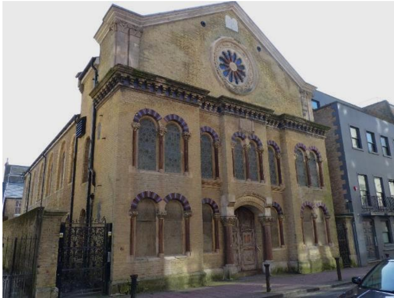
The Synagogue, Middle Street – Listed grade II*
