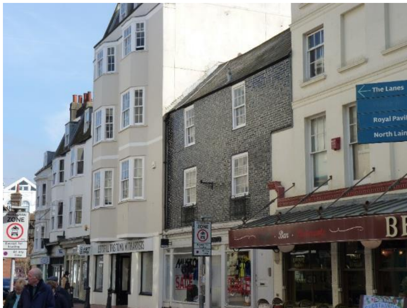
Building contrasts in Market Street including the glazed tiles at No.23
