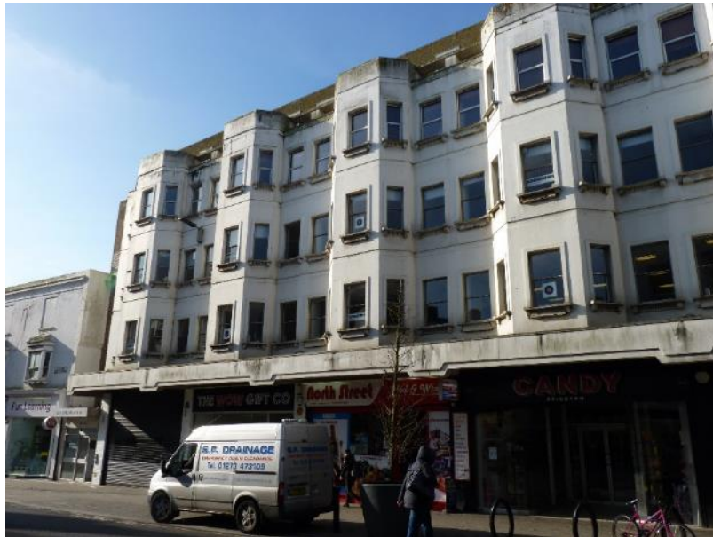
Nos.21-25 North Street
