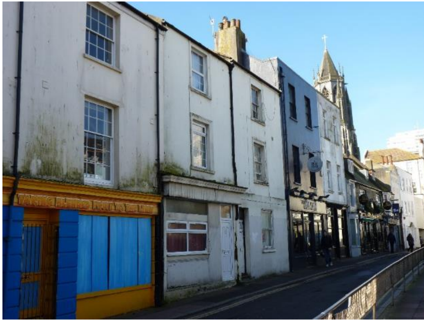
Boyces Street: Plastic windows and door at No.6
