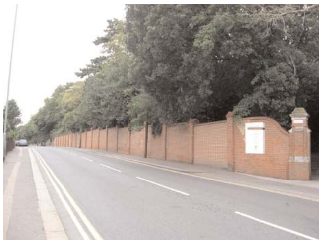
Fig. 7 - Loxdale frontage of Locks Hill
