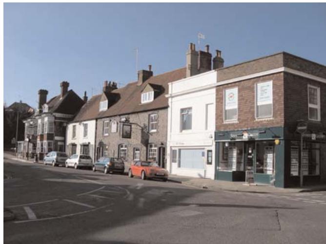
Fig. 15 West portion of the High Street
