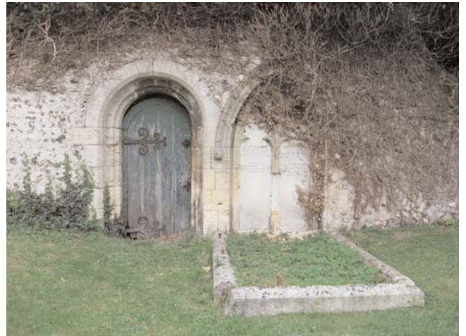
Fig. 3 - Doorway formerly giving access between church and Portslade Manor
