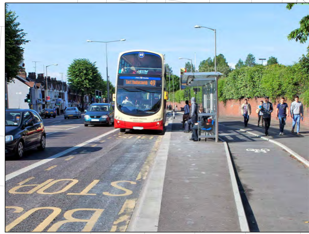
Image 2 - Example of floating bus stop
