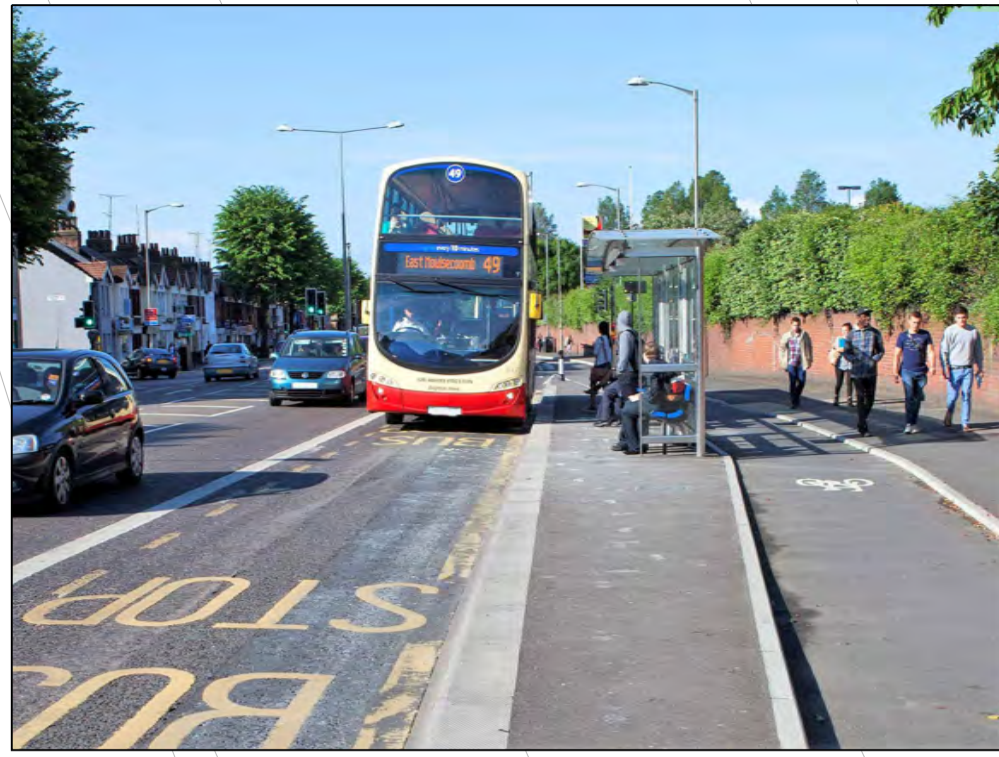
Image 2 - Example of floating bus stop
