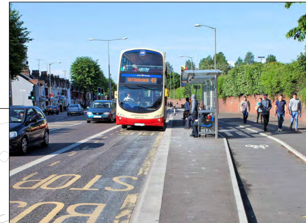
Image 2 - Example of floating bus stop
