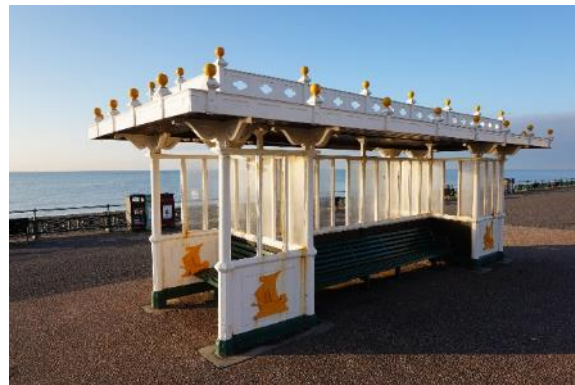
b) Grade II listed shelter
