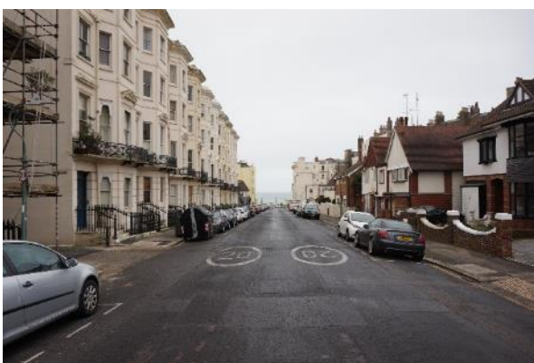
a) Holland Road (view to south)
