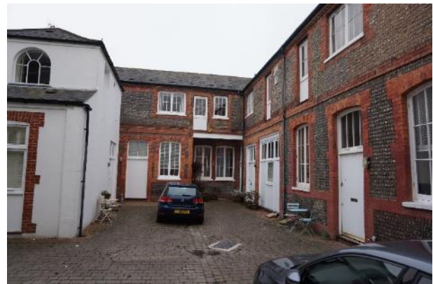
f) Flint and brick mews buildings, Goldsmid Mews
