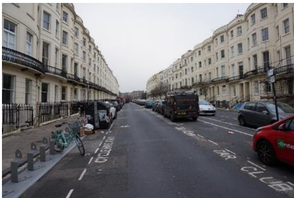
c) View to north, Brunswick Place
