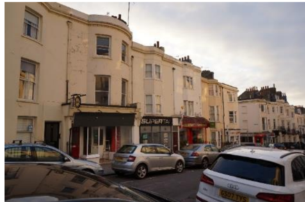
d) Nos 37-42 Waterloo Street (east side)
