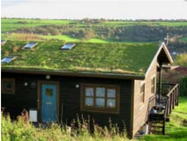
Figure 9 green roofs benefit biodiversity and provide ecosystem services, such as reducing storm water runoff
