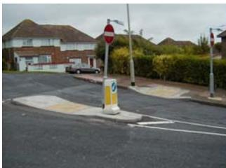
Where a formal pedestrian crossing is not justified these can be installed. They assist pedestrians by letting them cross the road in two stages. The restriction to the use of this measure is the width of the carriageway. It must be at least 7.8m wide to allow for the island and two lanes of traffic.
