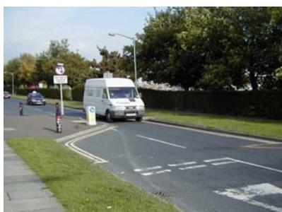
Chicanes and throttles are intended to reduce traffic speed by reducing the available carriageway width throughout a short length. Chicanes introduce a physical deflection into the vehicles' horizontal path, thereby further reducing the vehicle speed. Throttles narrow the road, frequently to provide a safe crossing point for pedestrians, sometimes in conjunction with a speed table.
