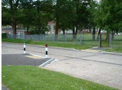
At some road junctions visibility is often reduced because of the shape of the road or because of parked cars. Building out the kerb into the carriageway can help solve this problem. It provides protection for motorists emerging from a side road as they can safely pull further out to see, and be seen. Pedestrians are similarly protected, have more space to stand and can also see and be seen better. Cars are forced to park further from a junction or crossing point.
