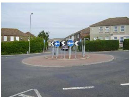
Standard roundabouts are intended to assist at a junction where there is a heavy right turning movement. They work best where traffic flows on each arm are reasonably well balanced and they allow traffic to flow comparatively freely.
