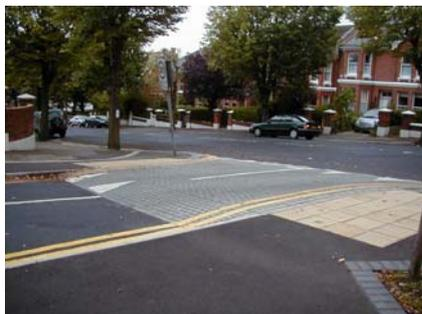
A junction entry treatment is placed across the carriageway of the minor road at a road junction. The object is to show motorists that they are leaving a main road and entering a residential area and to raise the priority for pedestrians crossing the junction. This treatment often has a speed table, kerb build out and gateway features.
