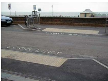
Tactile paving is now used at all new zebra and pelican crossings to help people with impaired vision. Similar tactile paving is also used at many ramped crossing points. Many single pelican crossings have audible signals, as well as the green man signal, to indicate when it is safe to cross the road.
