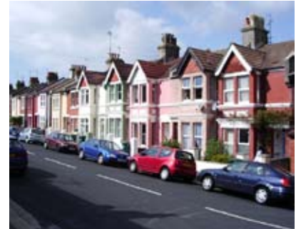
Edwardian terraced housing with bay windows
