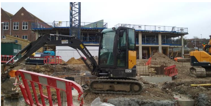
Work underway at Hobby Place
