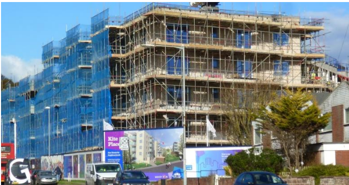
West block under construction
