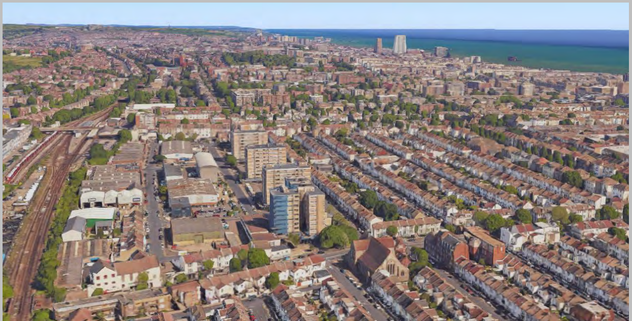
Aerial view of area looking south-eastwards towards Brighton
