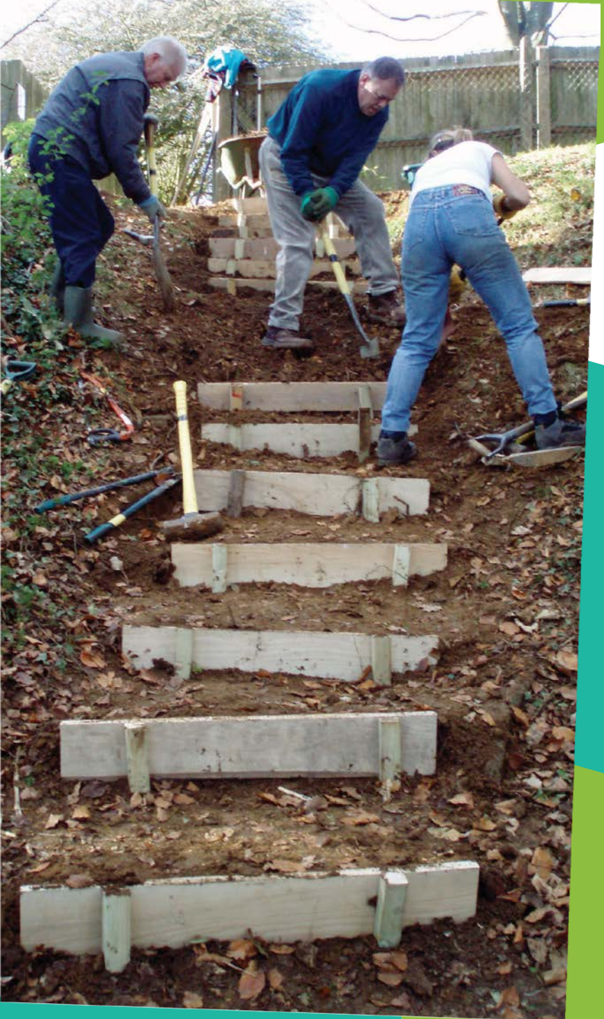
Step Installation Three Corner Copse
