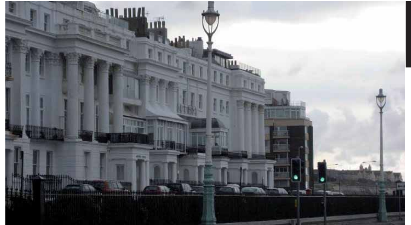
Fig 38: Detail of east end of Arundel Terrace showing the visual relationships with 'De Courcels'.
