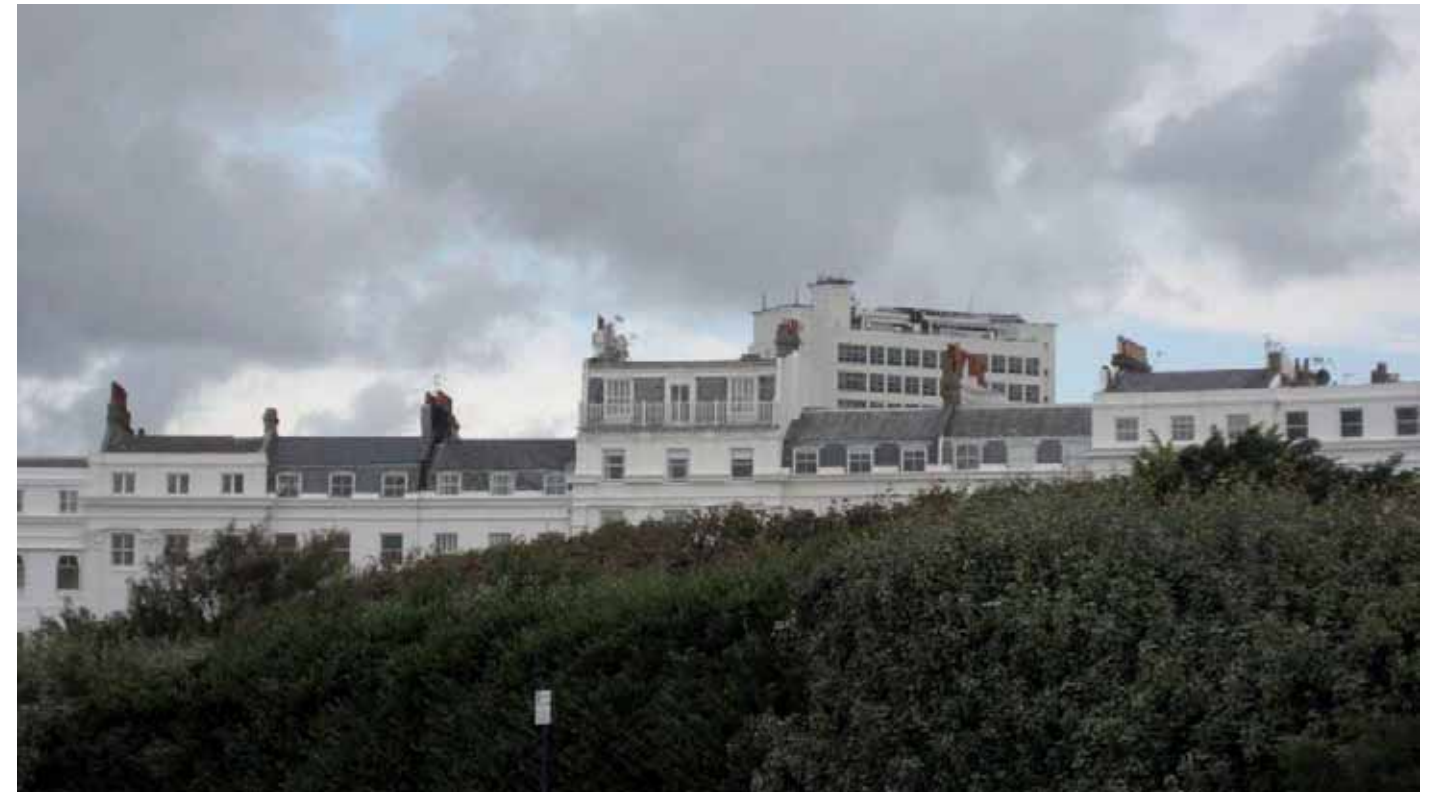
Fig 41: View from Marine Parade with the hospital Kemp Tower forming a backdrop to the centre of the west quadrant of the Crescent.
