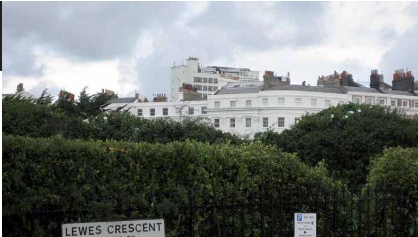
Fig 40: View from west side of crescent, with the Kemp Tower hospital forming a substantial backdrop to the Cubitt House (No.17).
