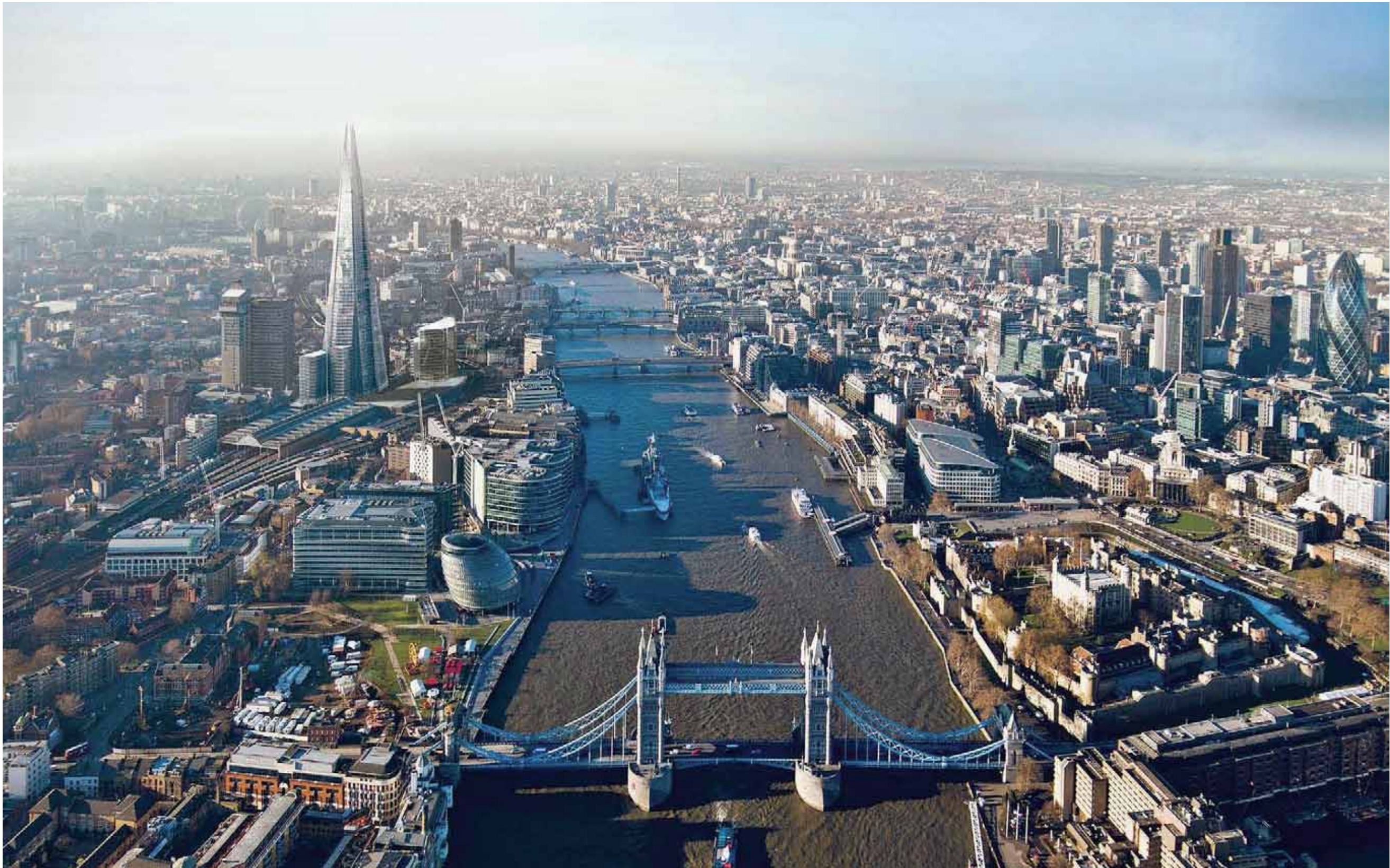
Fig 9: Showing an aerial view of the City of London, the Tower of London, Tower Bridge, More London and the London Bridge Station cluster of tall buildings, including a montage of the Shard of Glass, now under construction. In views from the former Royal Mint Yard, the Shard will be seen rising beyond the central silhouette of the Tower.
