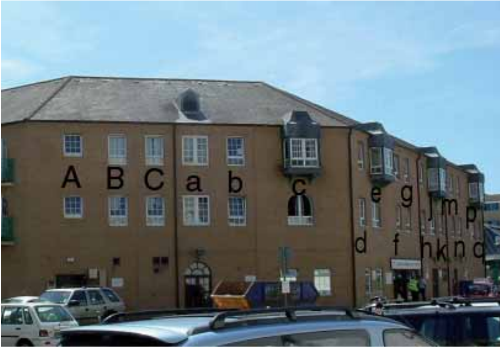
Figure A2. North west and west (to right of picture) faces of the Octagon building. The west side faces the current Asda (proposed Cliff site) directly. Window letters correspond to those in tables A2-A4. The capital letters denote residential windows; windows labelled with small letters (including the whole of the west face) light offices.
