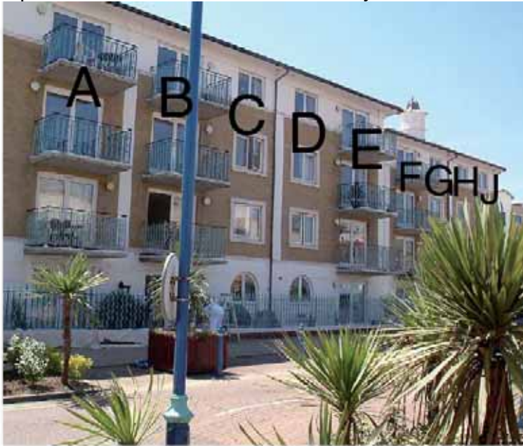
Figure A1 The north side of Neptune Court facing the Inner Harbour site. Letters refer to window locations in table A1.
