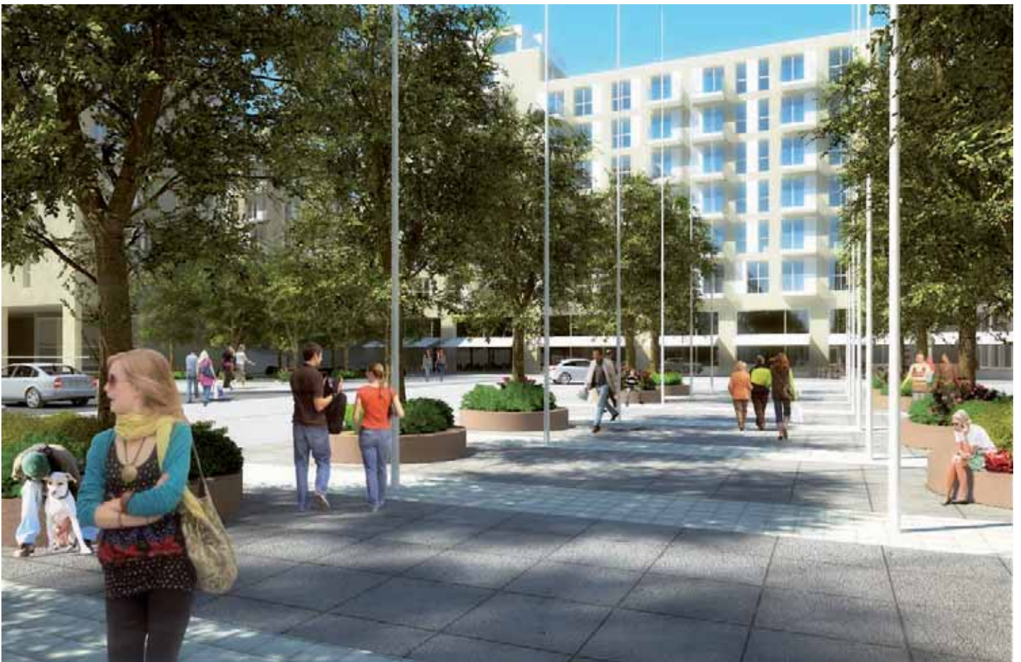
Harbour Square looking north towards the cliff building
