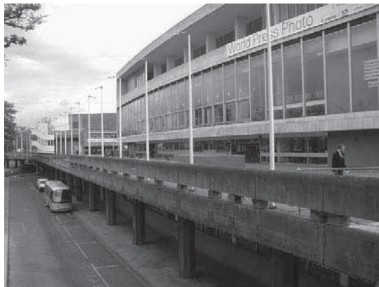
The existing building
