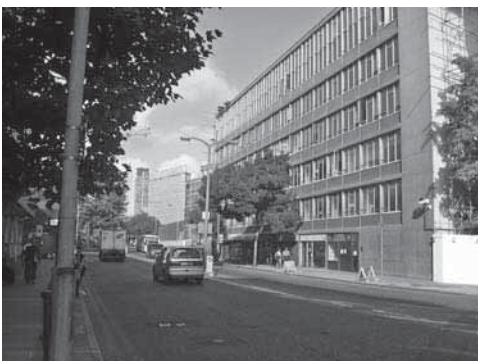
The existing building
