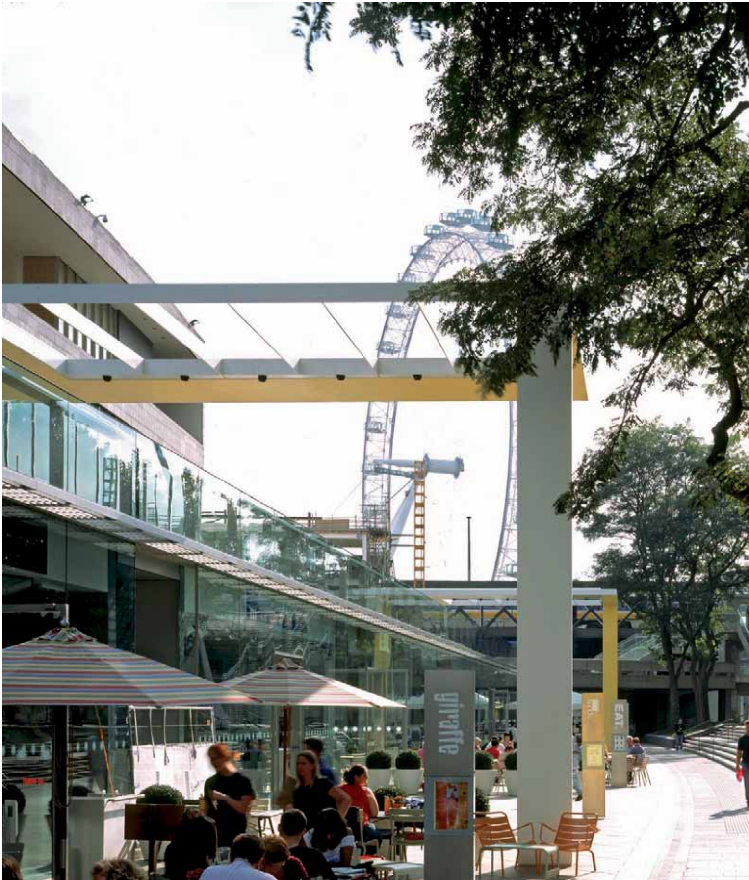
The Royal Festival Hall, part of the transformation of the South Bank carried out by Allies and Morrison in 2007
