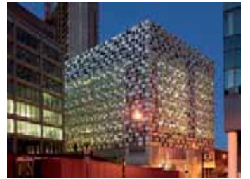
Multi-storey car park, Sheffield
