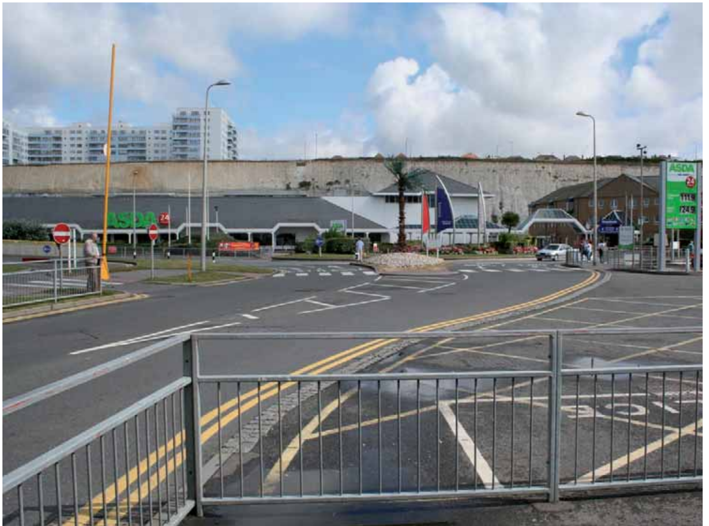
The view that greets the pedestrian at the bottom of the flight of steps as they leave the cafés and restaurants of the boardwalk
