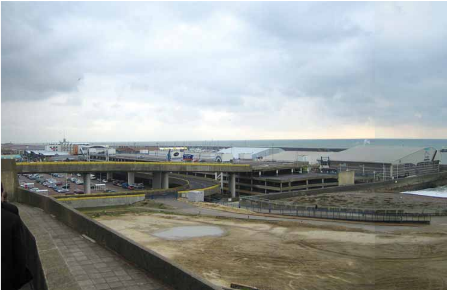
View across Black Rock site towards car ramp, car park and leisure sheds
